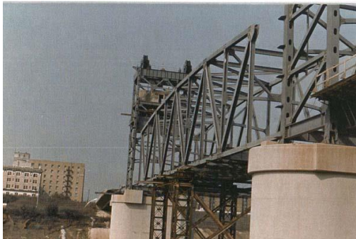
RED RIVER BRIDGE - ALEXANDRIA, LA
