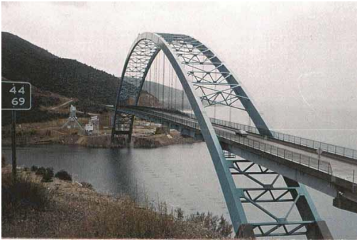
ROOSEVELT LAKE BRIDGE, ARIZONA 1991 AISC PRIZE BRIDGE WINNER - LONG SPAN
