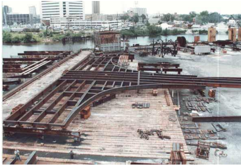
T-RAMP INTERSECTION BRIDGE - HOUSTON, TX
